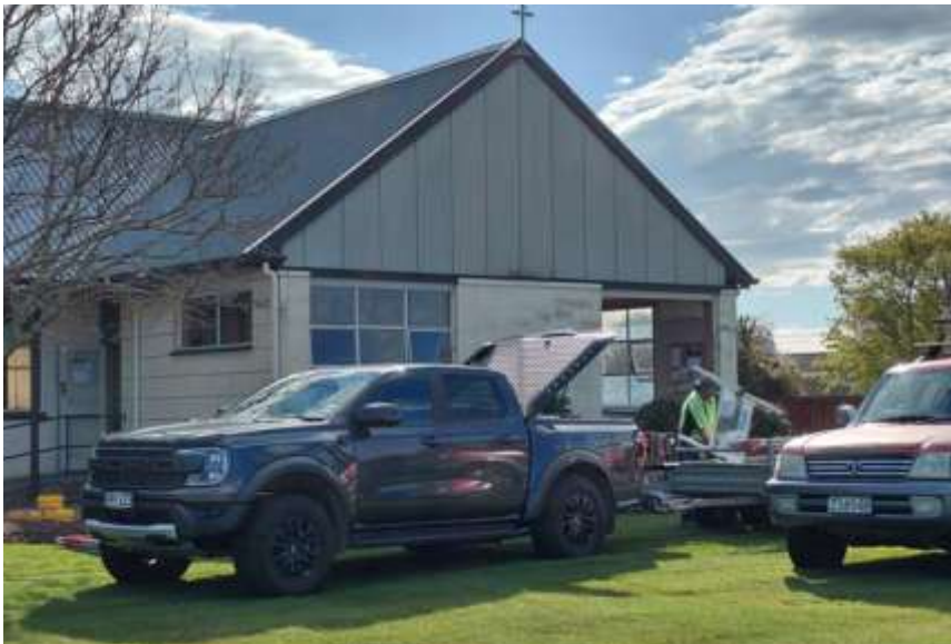
Installation of double-glazed windows in the offices at St Stephens
